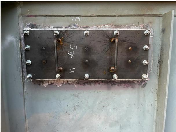
**Figure 2.** Example of access door install in progress.
