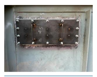
Figure 2. Example of access door install in progress.
